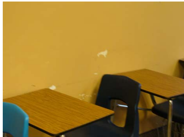
Typical Furniture Damage to Walls
