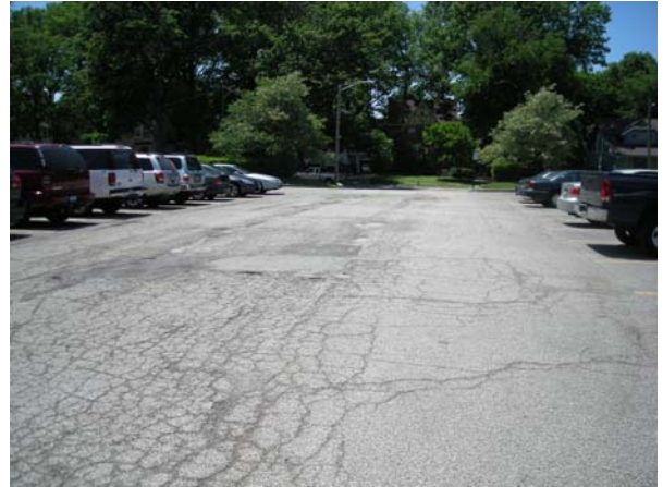
Damaged Asphalt in Parking Lot
