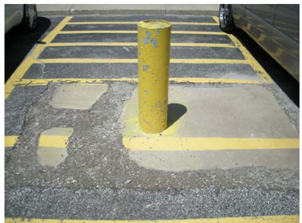
Damaged Concrete in Parking Lot
