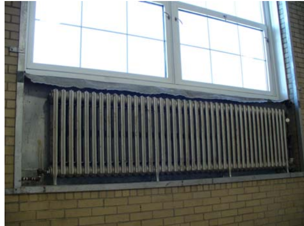
Typical Sill Condition at Gymnasia
