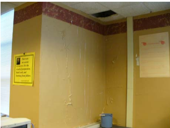
Water Damage in Technology Classroom
