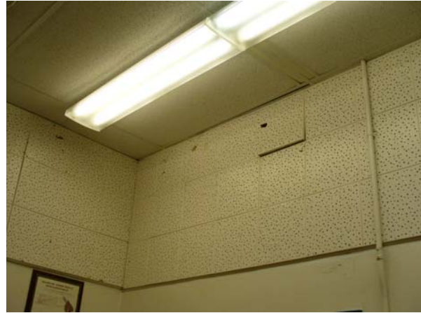
Acoustic Wall Treatment at Orchestra Room
