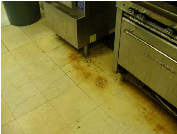
Damaged VCT in Kitchen
