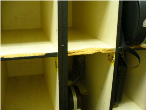
Deteriorating Music Storage Casework
