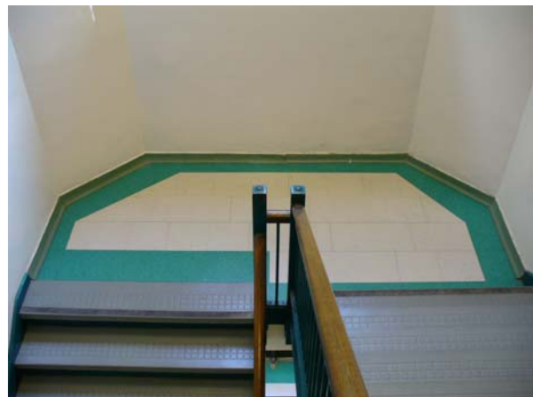
Typical Stairwell VCT Pattern
